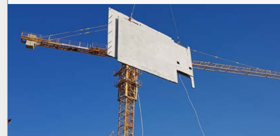
Off-Site Construction 시공
