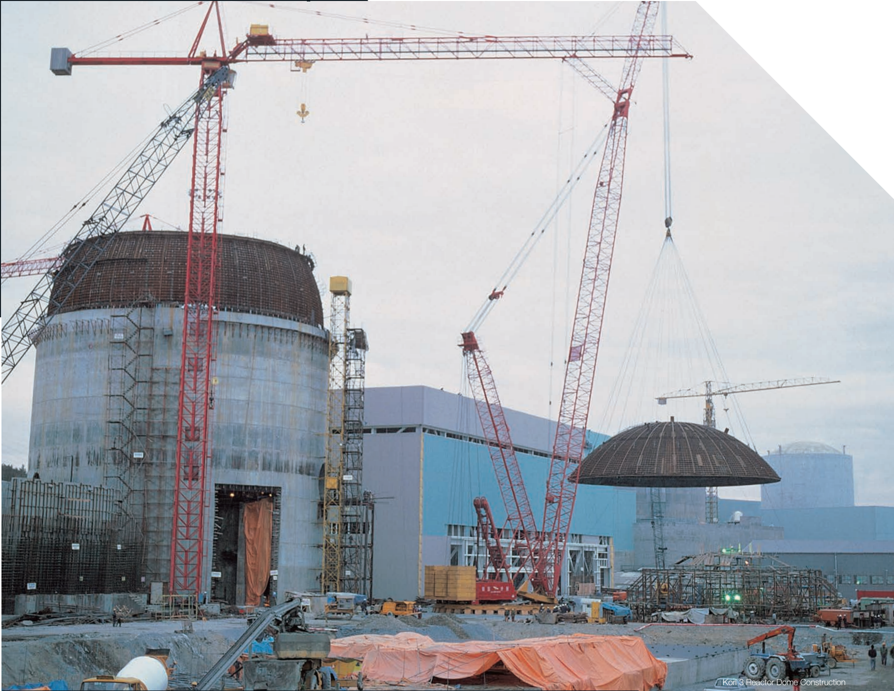
Kori 3 Reactor Dome Construction
