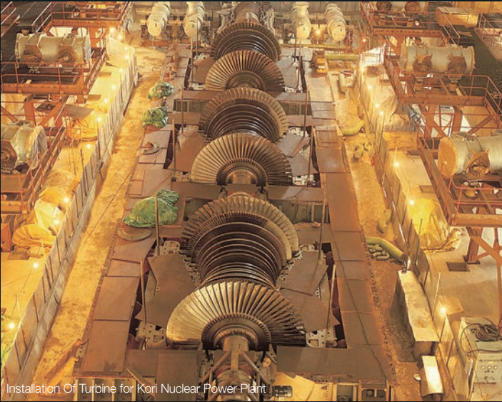
Installation Of Turbine for Kori Nuclear Power Plant
